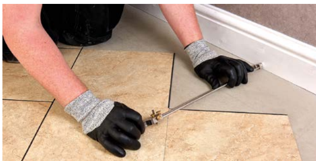
Figure 10 Cutting the tiles using a scriber (diagonal cut)
